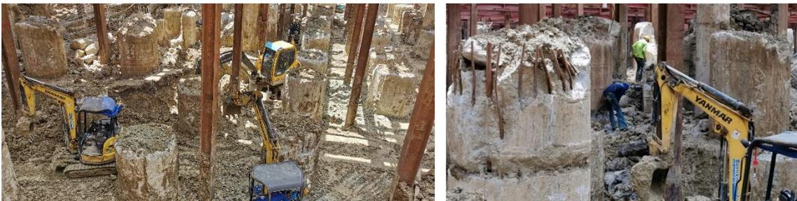
(Pile caps before cutting and shredding into aggregate at One Bangkok)
